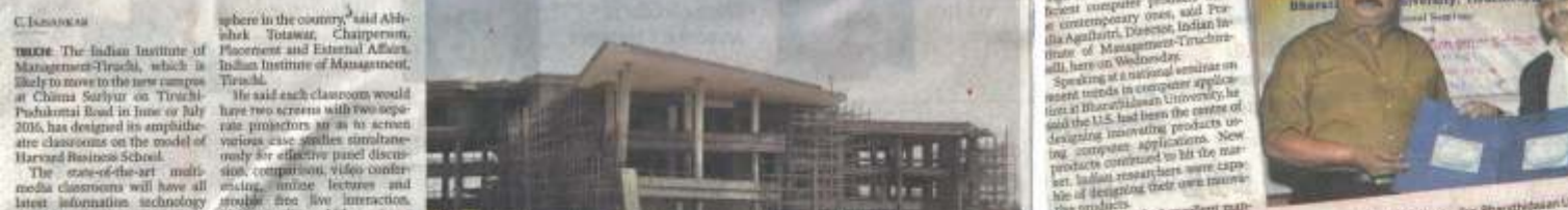
Classrooms of various sizes being constructed at IIM Tiruchirappalli.
